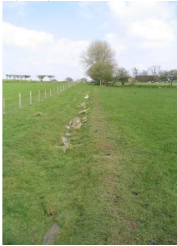
The stone-lined gully, used to house flat-rods
