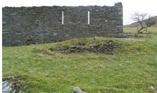
Southern elevation of Nant-y-Maes, showing ventilation slits.
