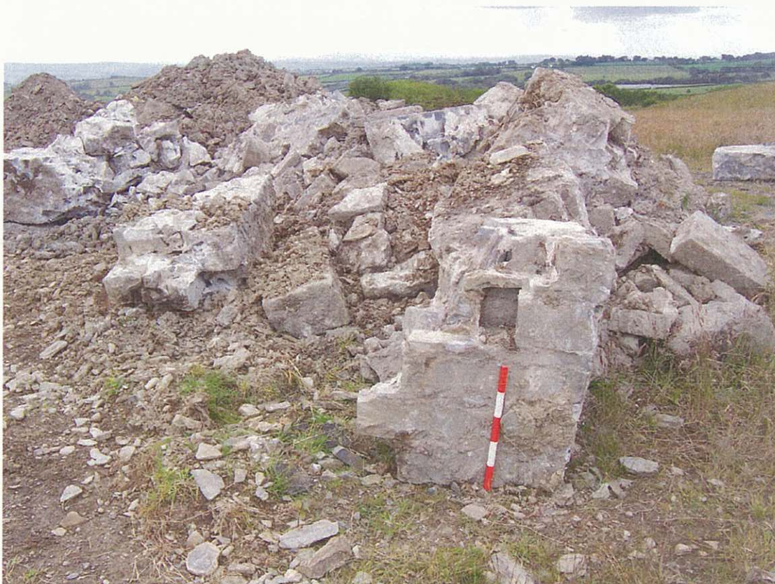
Photo 5: Masonry from collapse, original socket for timber. Scale 0.5m
