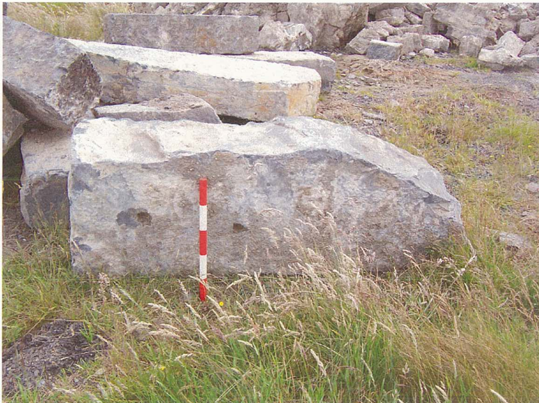
Photo 10: Massive stone with two bored holes, only the left goes through stone. Stones now at depot
