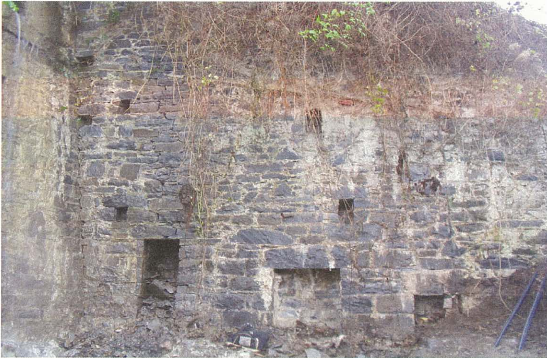
Photo 9: The north revetment wall of slipway showing the various features in the wall and the roof line scar. View NW
