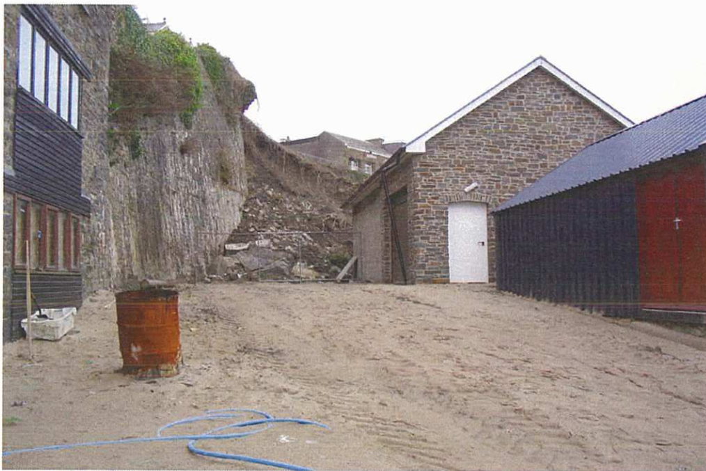
Photo 10: North end of slipway after collapse of northern revetment
