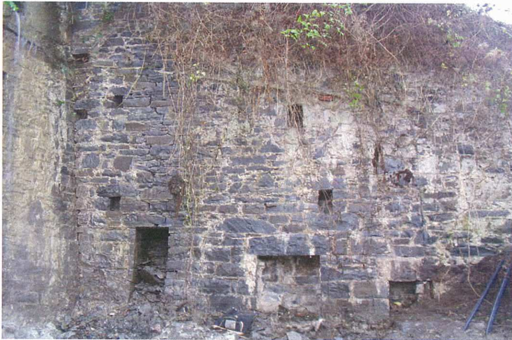
Photo 3: The north revetment wall of slipway showing the various features in the wall and the roof line scar.
