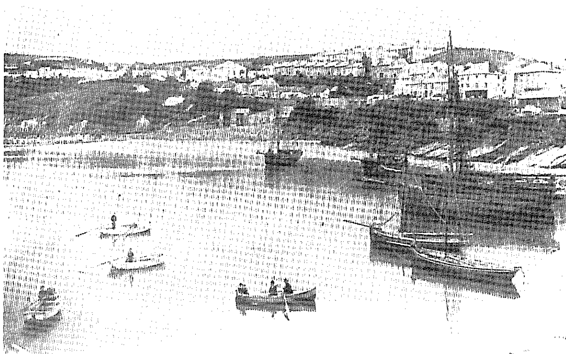
Plate 1: Photograph c. 1880, showing the Patent Slipway in the background. The building at the north (right) end of the slipway would presumably have housed the winch mechanism. Also note the vertical lines along the slipway. These may be part of the cradle for supporting ships on the slipway.
