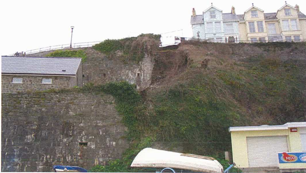
Photo 9: North end of the slipway after collapse of the north revetment wall.
