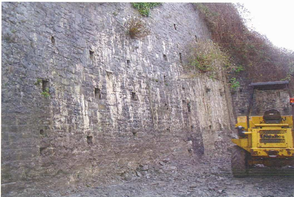
Photo 4: The west revetment wall of the slipway showing seep holes and other features north of the warehouse.
