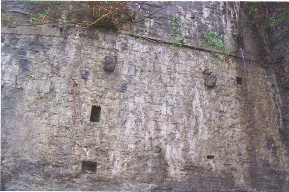
Photo 5: North end of the western revetment wall showing corbels, roof scar and other openings.
