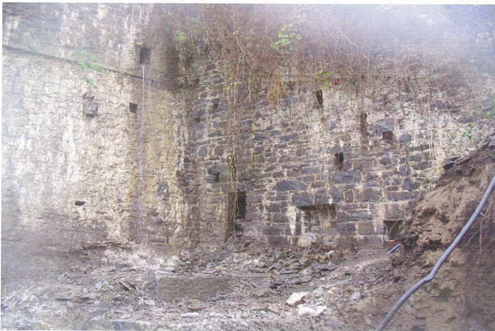
Photo 6: North end of slipway. Note the exposed foundations for the winch mechanism.
