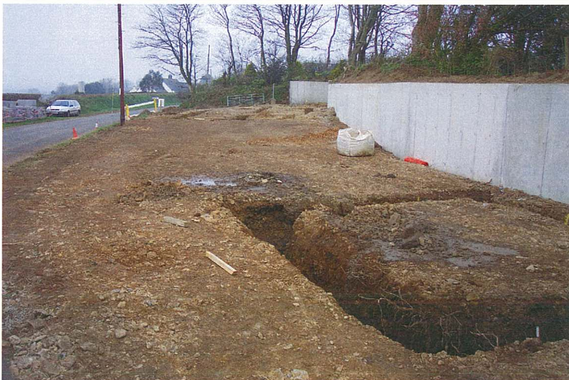
Photo 1: Site as cleared and footing trenches excavated. Garage footings in foreground. View W
