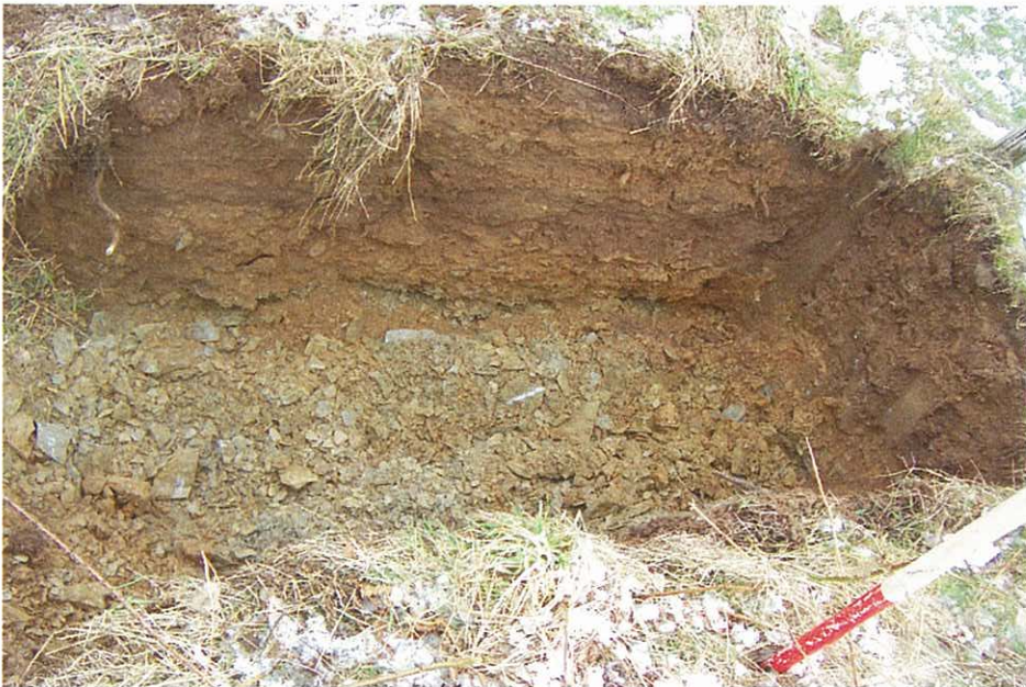
Photo 2: Cut for 'stay' for easternmost pole
