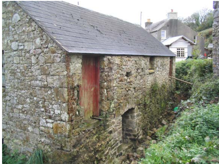
A large trench at the rear of the mill building has recently been excavated, and it is of some concern that this may threaten the stability of the building.
