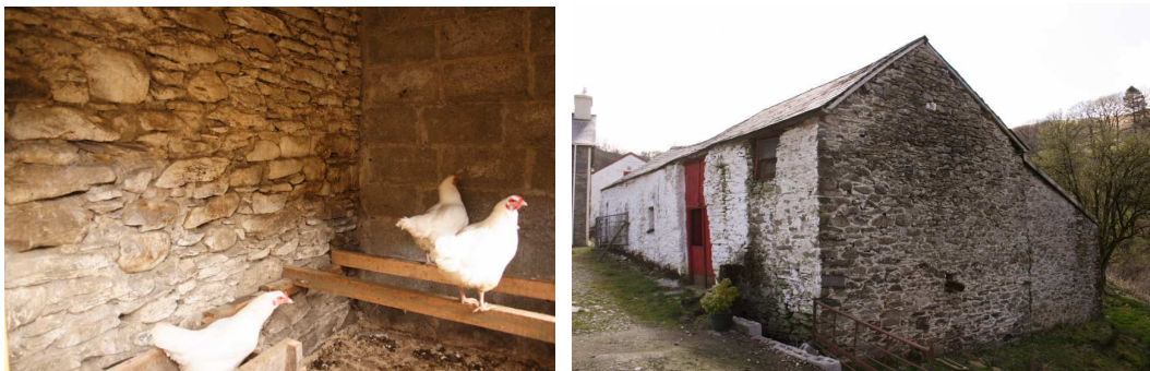
Unpainted masonry within the chicken-house and on the threshing barn gable end.
