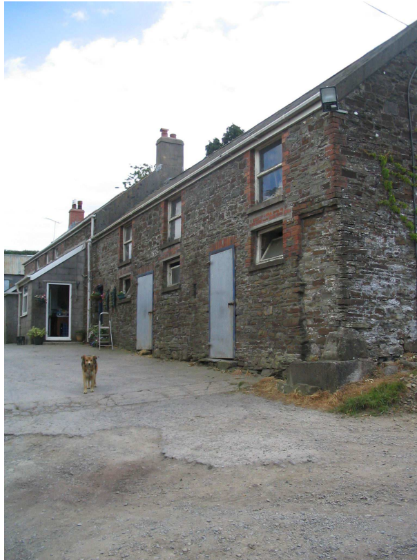
North elevation of farmhouse and barn (51025), showing brick insertions.
