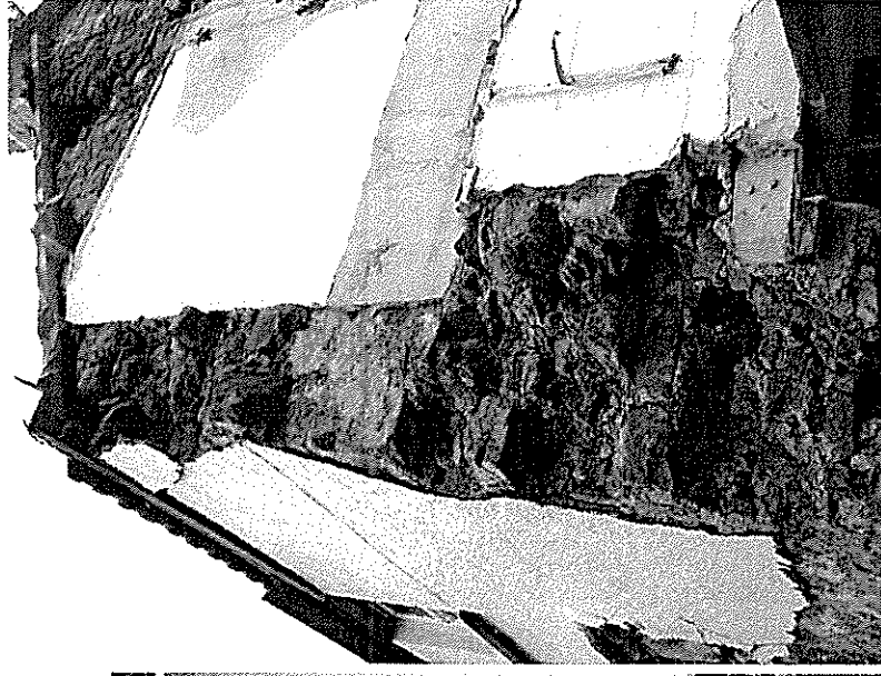
Photo 4: Showing faced stonework of vertical window jamb in truncated wall end.
