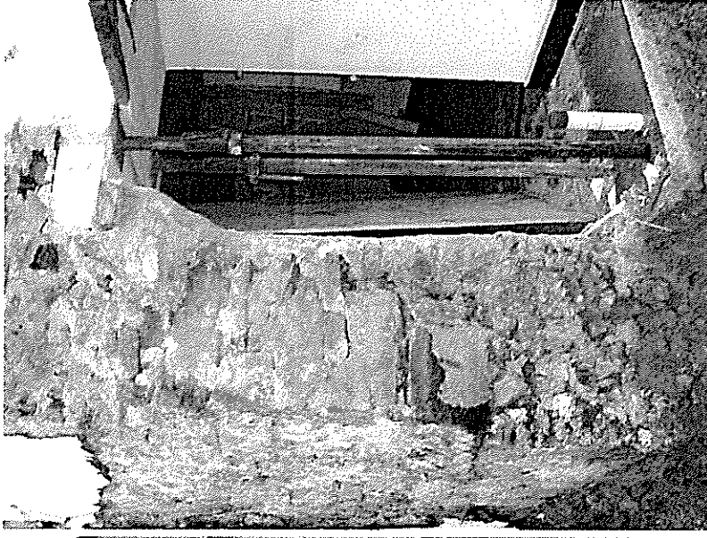
Photo 3: Truncated wall remnant showing 'pillar' of natural below stone footings, faced with rendered stone rubble. Note faced stonework of vertical window jamb.
