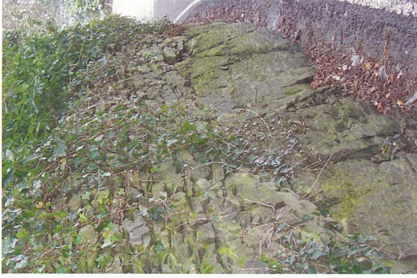
Photo. 22: Wall built upon bedrock.
