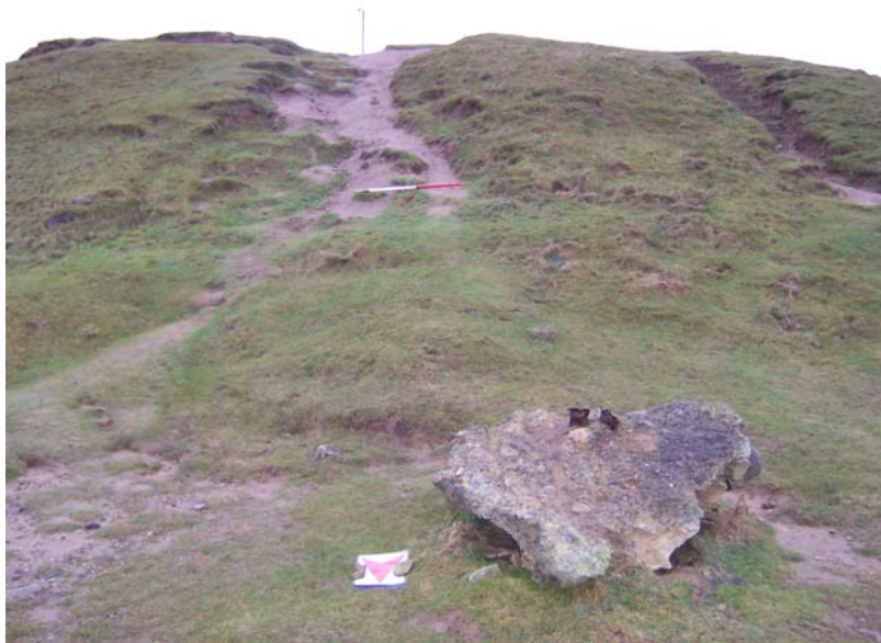
Plate 4: Visitor erosion is having a significant impact on the protective earth mound of the St. Govan's Head Observation Post (PRN 33454), despite the provision of purpose built steps (on the right). This mound is also suffering from severe wind erosion and burrowing animals.
