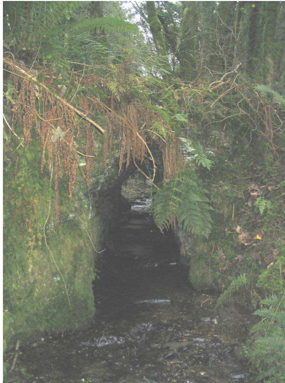
Prn 50020 – a fine stone built culvert with a corbelled roof channels the Gloyn just below the entrance to Cwmgloyne mansion.
