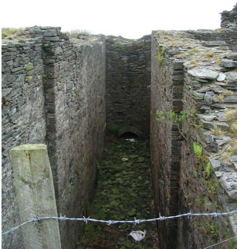
The wheel-pit, and its' south-eastern annexe.
