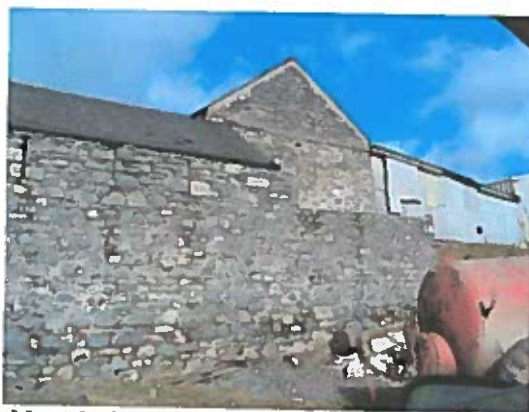
Cowshed on south side of foldyard, showing ventilation slits and gable end of carthouse with mortar scarring.
