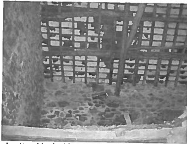
Inside the carthouse showing 'torching' which is a distinctive feature of the roofs at Mynydd Gorddu
