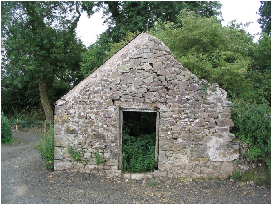
The masonry of the north gable wall is unstable, particularly above the doorway.
