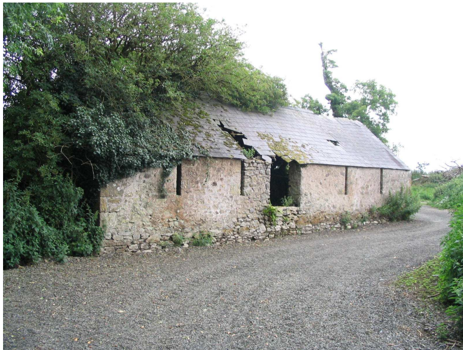
The cow shed at New Shipping farm, this building is threatened by encroaching vegetation and is no longer weatherproof
