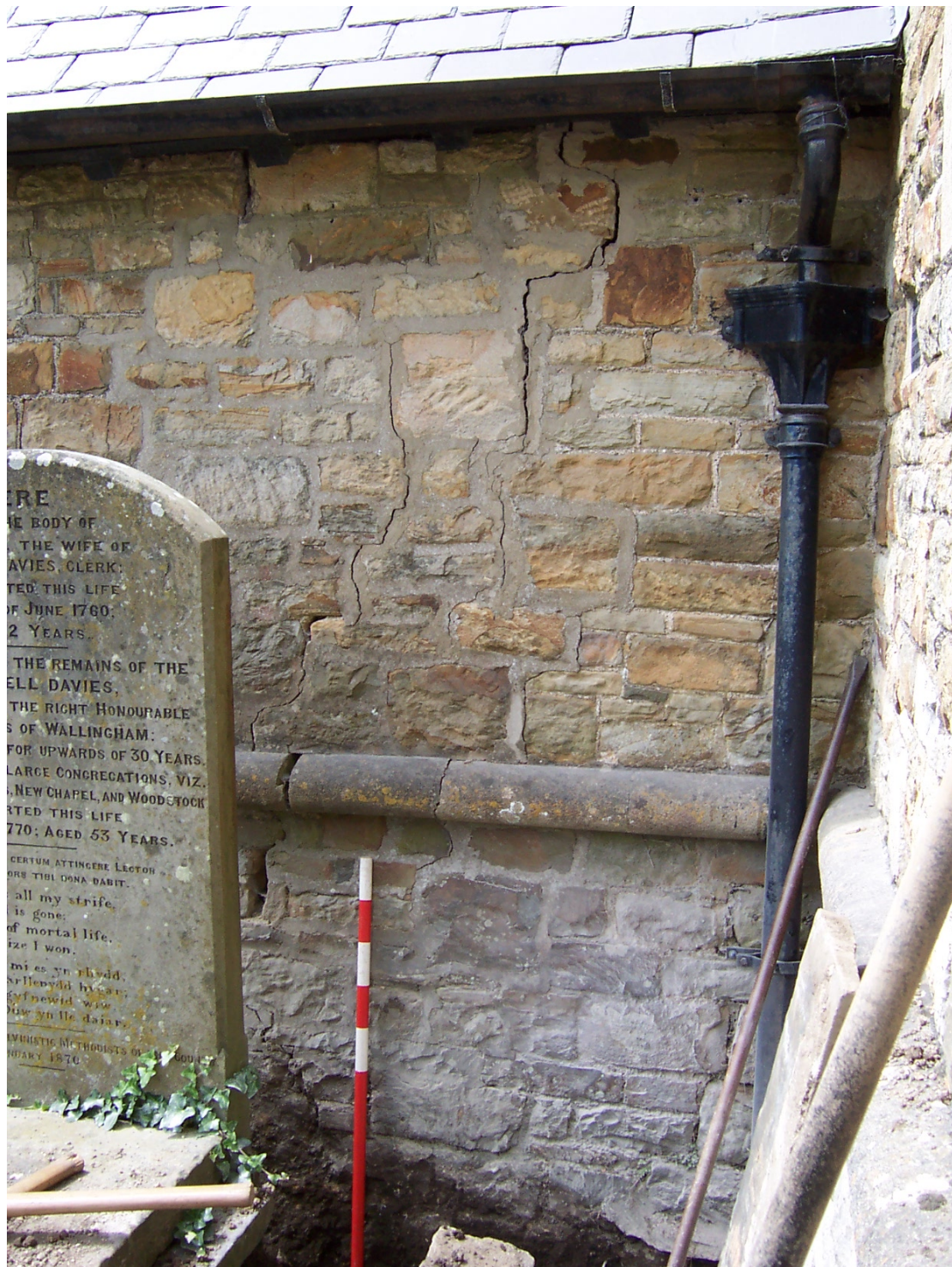
Photo 1: Subsidence crack on east side of porch. View W. Scale 1m
