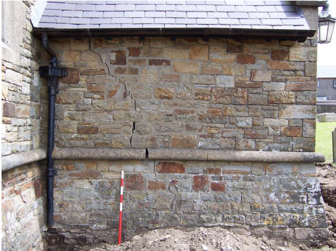
Photo 2: Subsidence crack on West side of porch. View E. Scale 1m
