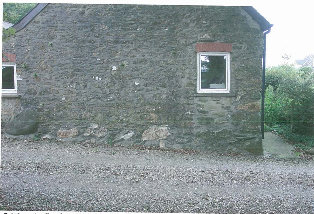
Plate 5 (above): South gable end of the holiday cottage (PRN 49140) which is probably a converted cowshed (PRN 49139). The base of the wall is constructed of large, irregular boulders and is very different to the rest of the wall. This may have been the stone base for clom walls.
