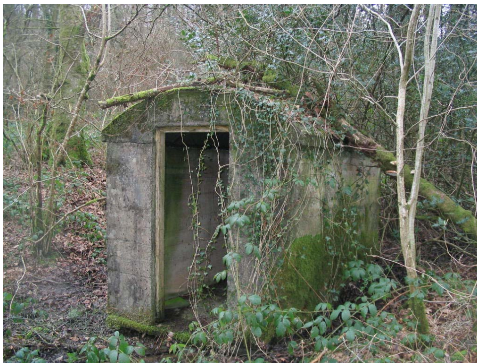
Plate 4 The explosives store, built of shuttered concrete and dated '1934'.
