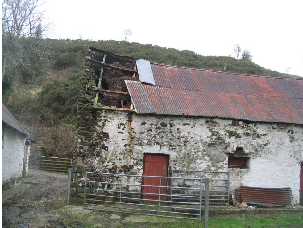
Plate 2 (above) West end of the cowshed, showing how the metal sheets have lifted, revealing surviving thatch.
