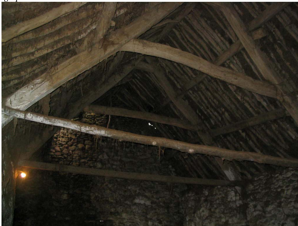
Plate 3 (below) Roof structure inside the cowshed. Note that the thatch in this building rests on whole, rough poles.
