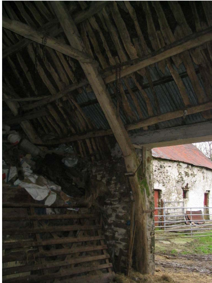
Plate 1 The interior of the barn, showing the scarfed cruck framing and an underthatch of split palings. The cowshed is visible through the doorway.
