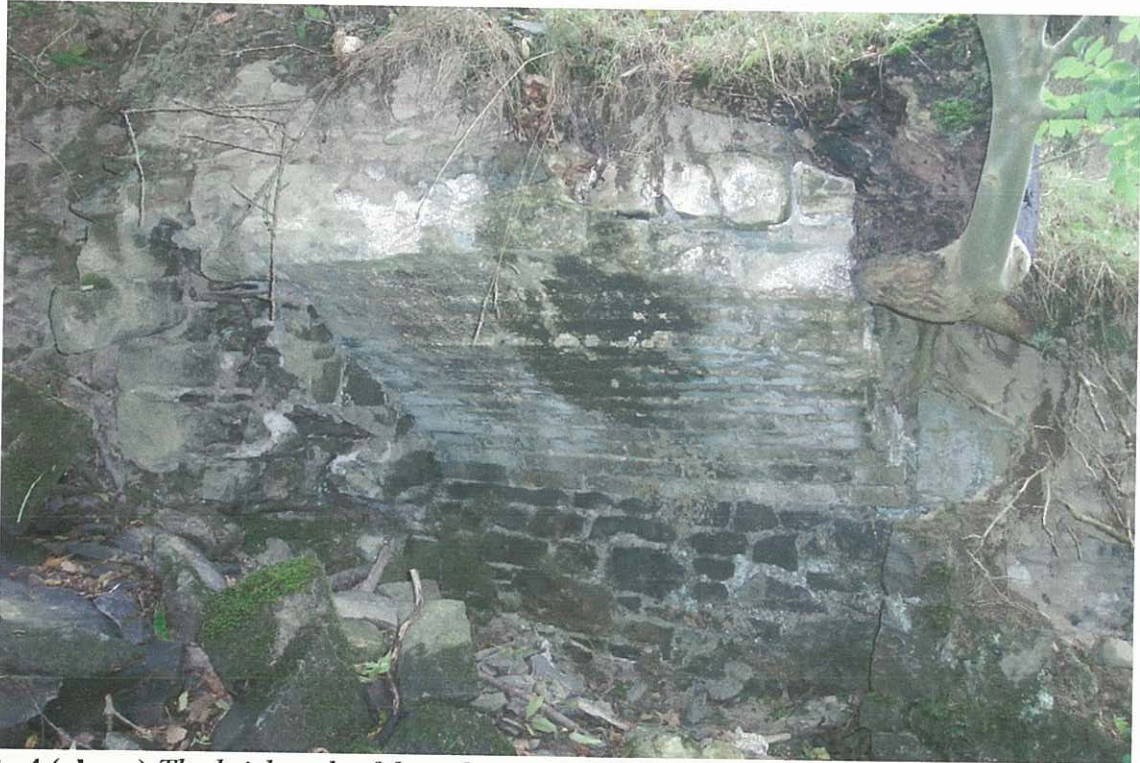
Plate 4 (above) The brick arch of the culvert which leads away from the pond (PRN 49180). New shoots from an old tree-stump are leaning heavily on the masonry.
