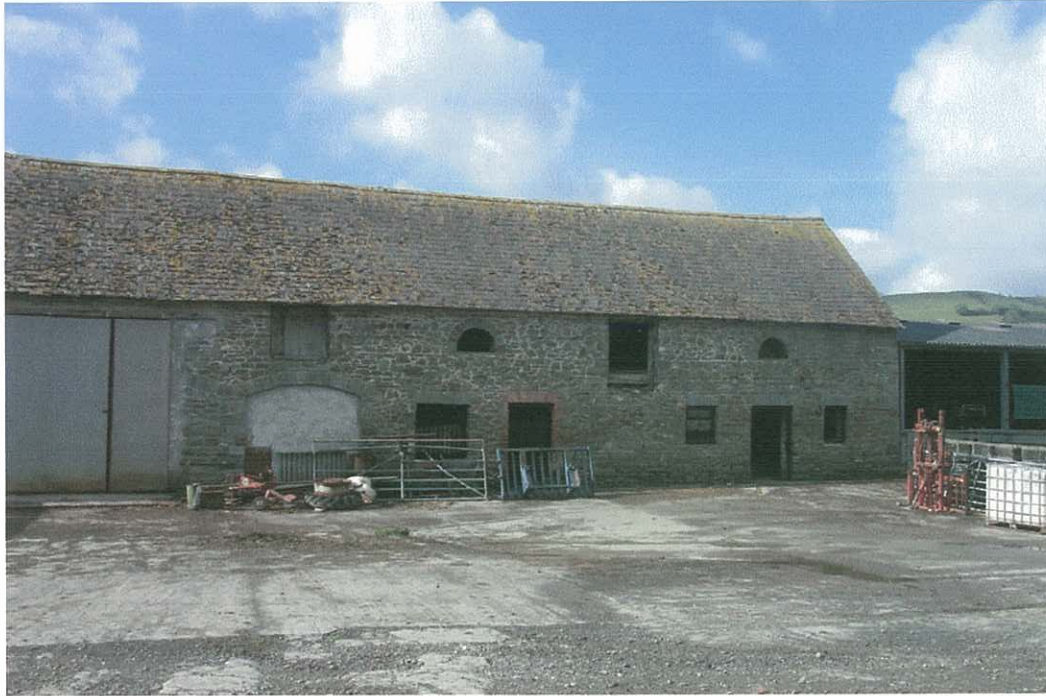
Plate 6 (above) The north-south range (north end) of the combination farm building, (PRN 49185). This houses stables and a now-blocked cartshed entrance. The modern doors (left of picture) cut through another cartshed entrance.
