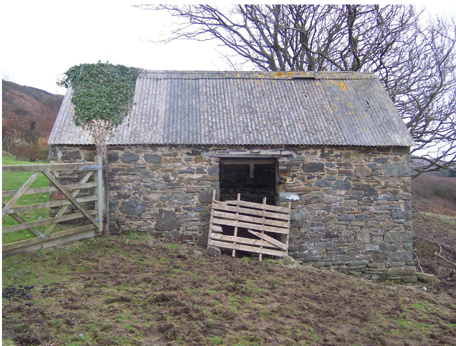
Prn 48712 – apart from the roof covering, this farm building appears to survive almost in its original form, with a stone flag floor internally.
