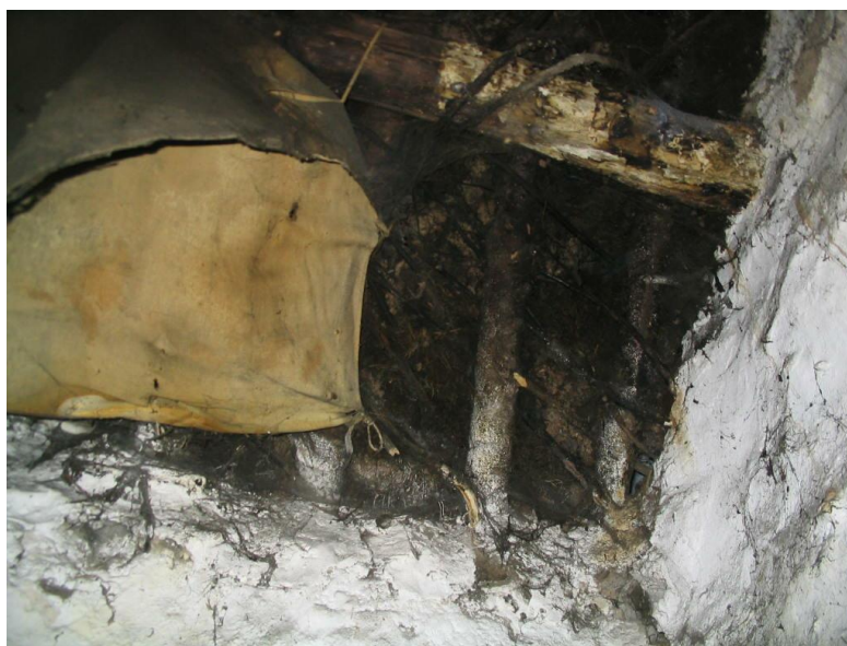
Plate 3. Part of the roof of Pen Rhiw cottage: close set poles taking the place of the rafters with an underthatch woven into them. The cloth would be in place to prevent parts of the thatch from falling into the room.
