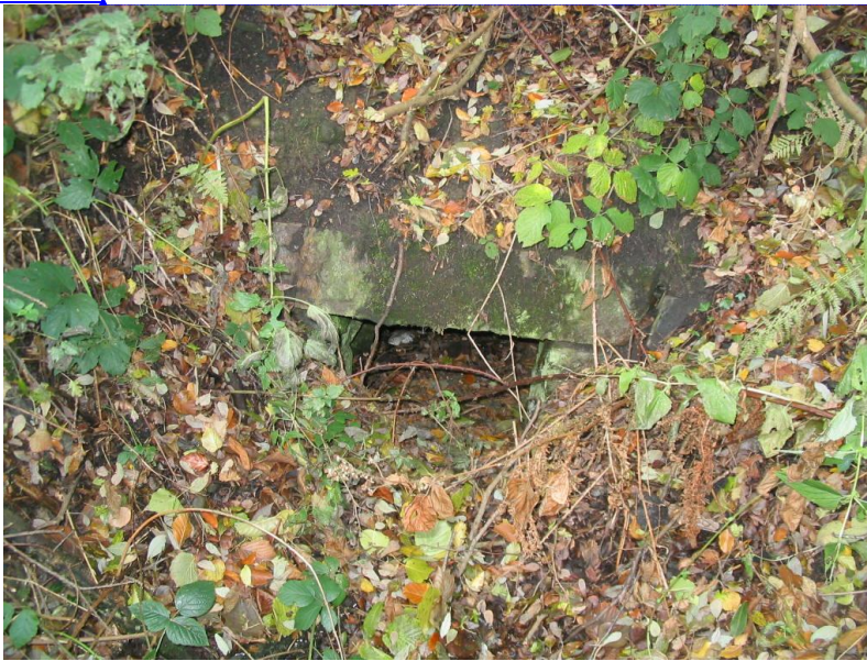
Plate 2 (below) A small, stone-built culvert passing under the embankment, now very blocked with silt and leaves.
