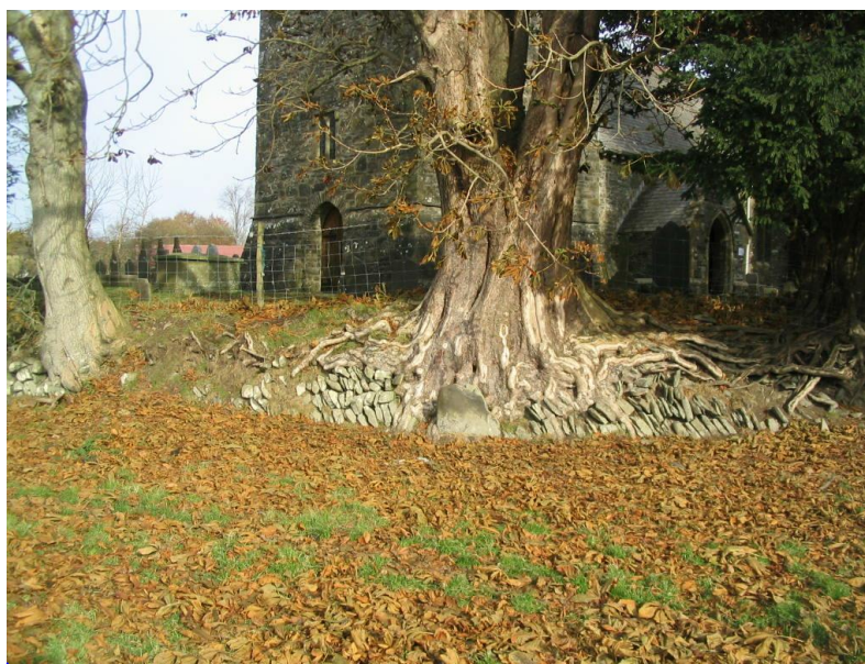
Plate 5. The boundary shared with St Peters Church, Llanybydder. Tree roots are pushing the stone facing off the bank, and there is little earth left that the stones can be set back into.
