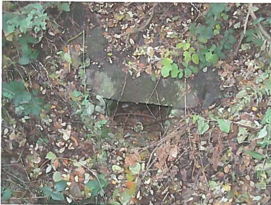
Plate 1 (above) The railway embankment, part of the dismantled Manchester-Milford line. Plate 2 (below) A small, stone-built culvert passing under the embankment, now very blocked with silt and leaves.
