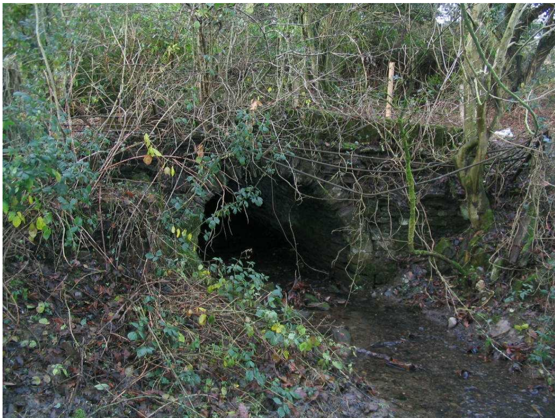
Plate 3 Bridge on Glanbrydan Park estate. The parapet is brick and was probably added after the original construction of the bridge.
