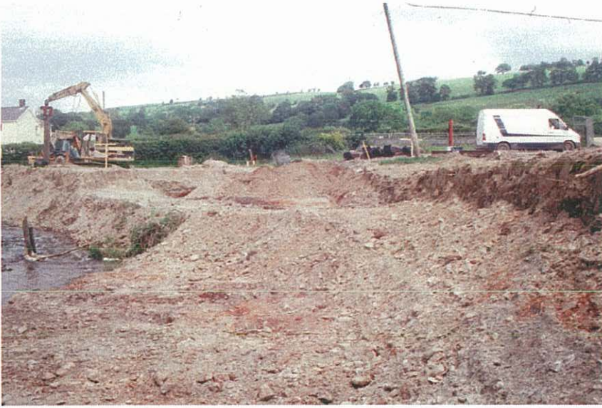
Photo. 4. Construction of the new bridge showing river gravels.
