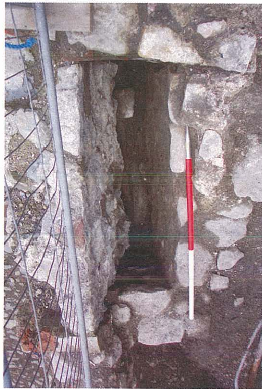
Photo 48: Area E. Blocked up barrel chute 134 in south wall of cellar 1.
