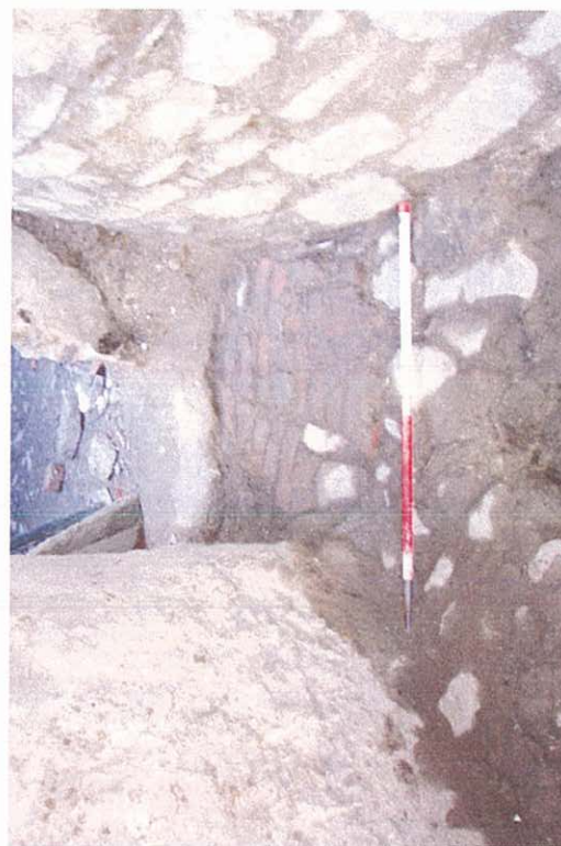
Photo 48: Area E. Blocked up barrel chute 134 in south wall of cellar 1.
