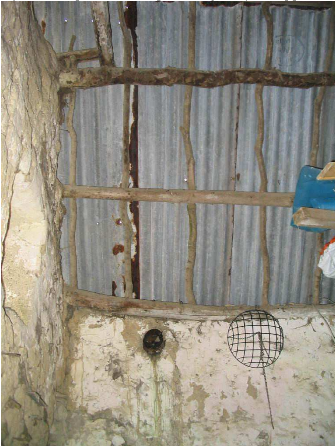
Below: Roof structure showing purlins made of whole branches set into the top of the wall. The rafters are spaced wide apart, originally to support thatch rather than slates.
