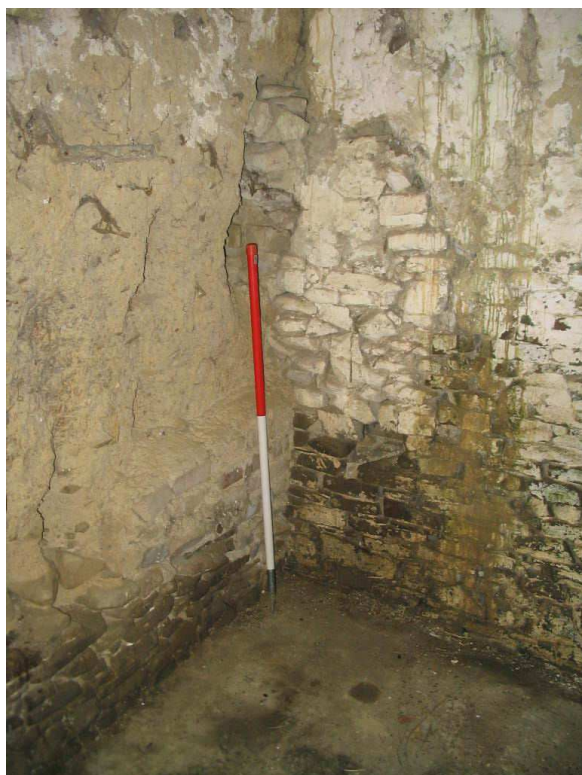
Above left: Joint between the northeast wall (right of picture) and northwest gable (left of picture).
