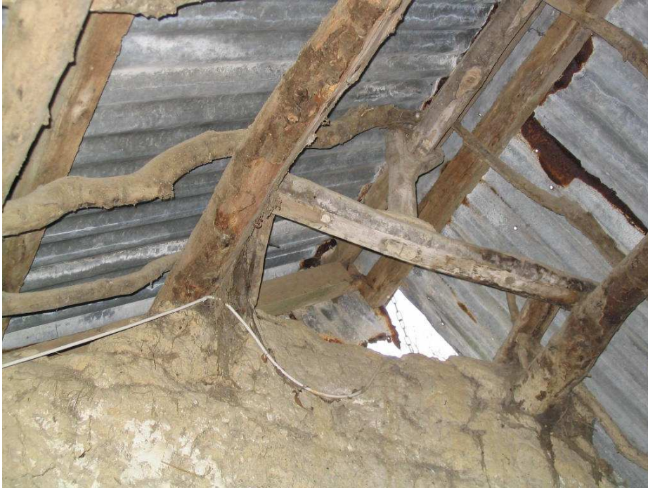
Improvised 'king-pin' supporting the ridge of the roof. This is constructed of a naturally forked branch slotted into a rough tie beam.
