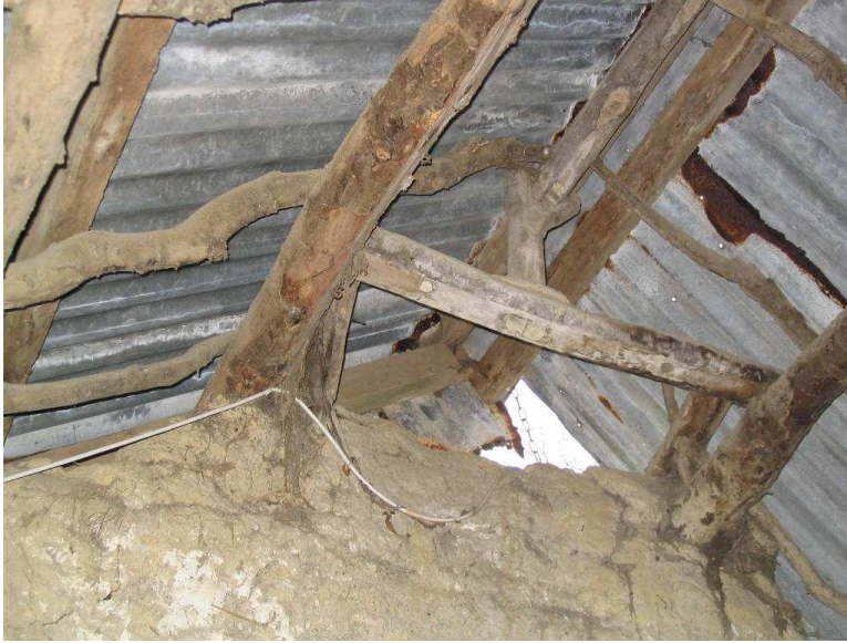
Above: Detail of the improvised 'king-pin' roof structure.
