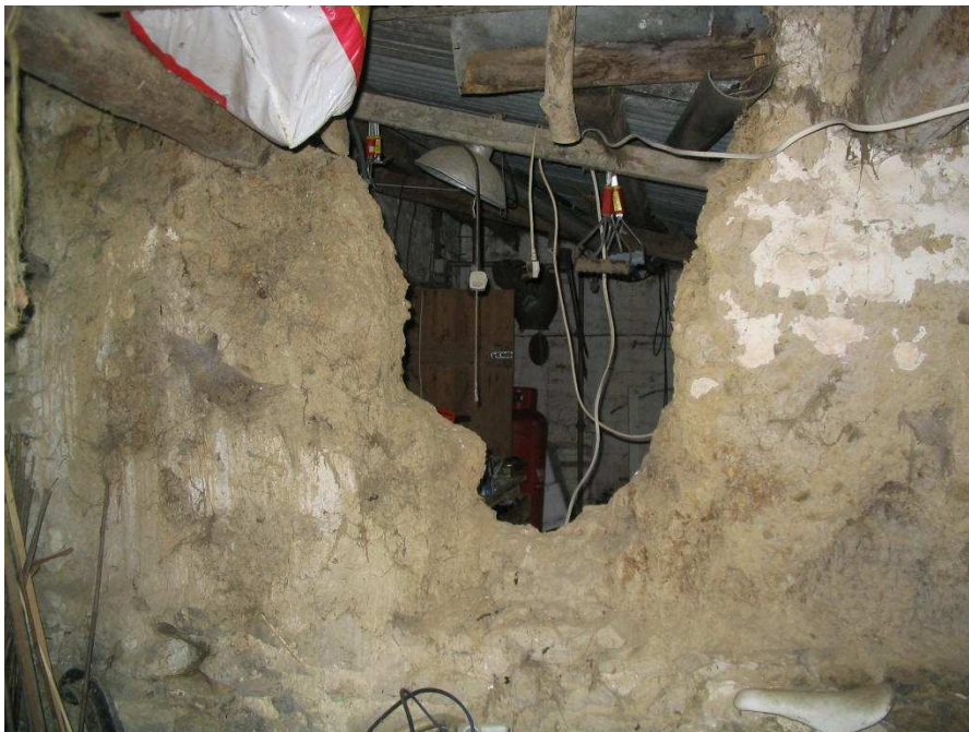
Part of the clom in the southwest elevation has been worn away by water run-off. This view is from the interior of the building, looking through the wall into the modern shed next to it.
