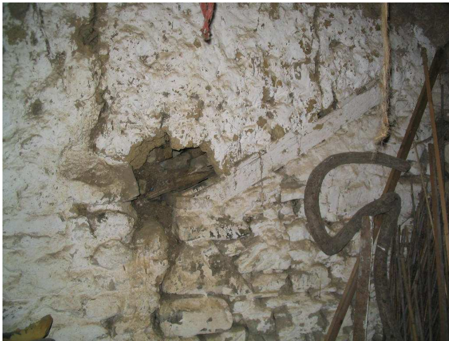
Sloping piece of wood, almost like the line of a lean-to addition, incorporated into the southeast gable wall.
