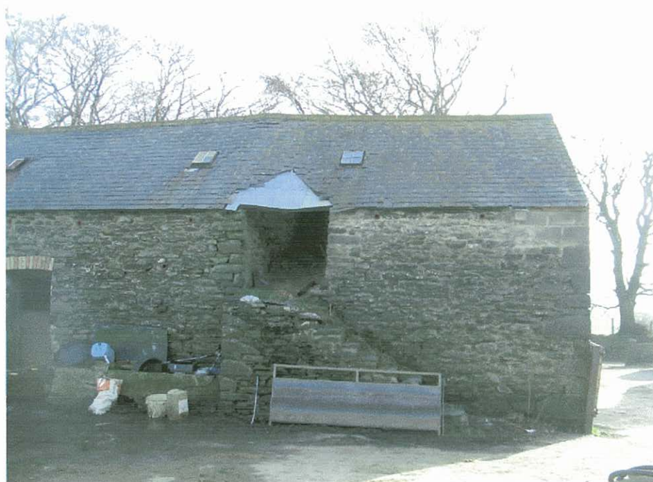
Plate 3 The south end of the combination farm building. The metal sheeting marks the shape of a dormer head, now lost.
