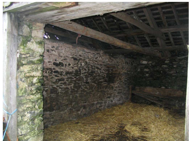
Plate 4 (right) Interior of one of the loose-boxes inside the building. The stone wall is an internal partition and the building would have had a hay-loft over.
