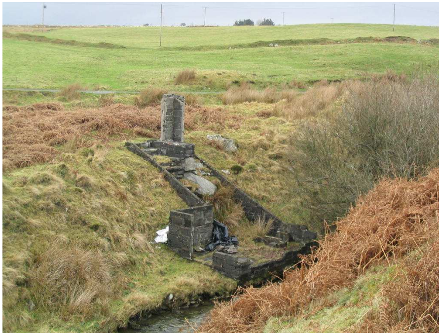
Plate 8 Remains of the housing for a turbine, next to a fast-flowing section of the stream.
