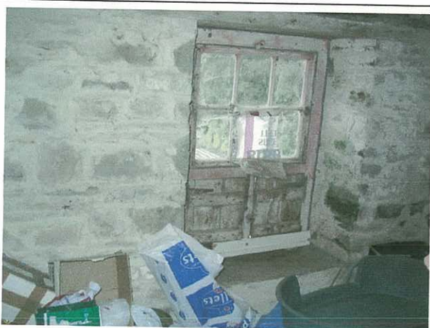
Plate 6 (left) Detail of the windows, showing six panes of glass above two wooden shutters.
