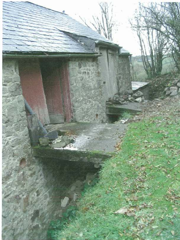
Plate 8 The south elevation of the barn, showing the gap between the building and the earth bank. Underneath the ramp in the foreground, the bank has slumped and earth is resting against the barn wall. The stone in that area comes from the largely collapsed retaining wall.
