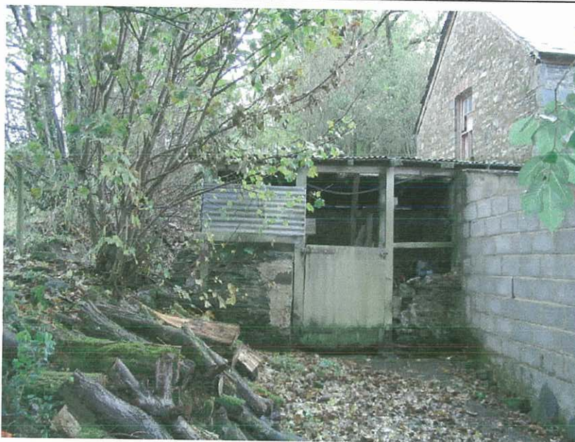
Plate 1 The pigsty against the east gable of the barn. The wooden door and corrugated metal walling were added when the pigsty was made into a stable. The breeze-block on the right of the picture is part of the modern car-port and shed, added against the north elevation of the building.
