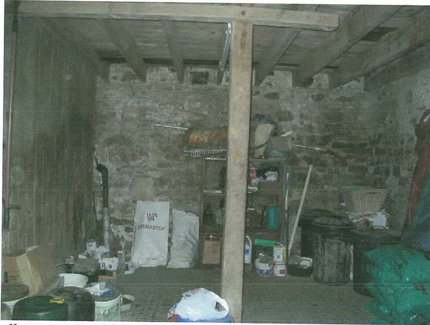
Plate 4 The well preserved stables which would have housed two working horses. Although the partition between the stalls is now gone, the upright wooden post marks its position. The wooden wall to the left of the picture forms the side of the feed/tack-room. Note the original stable floor.
