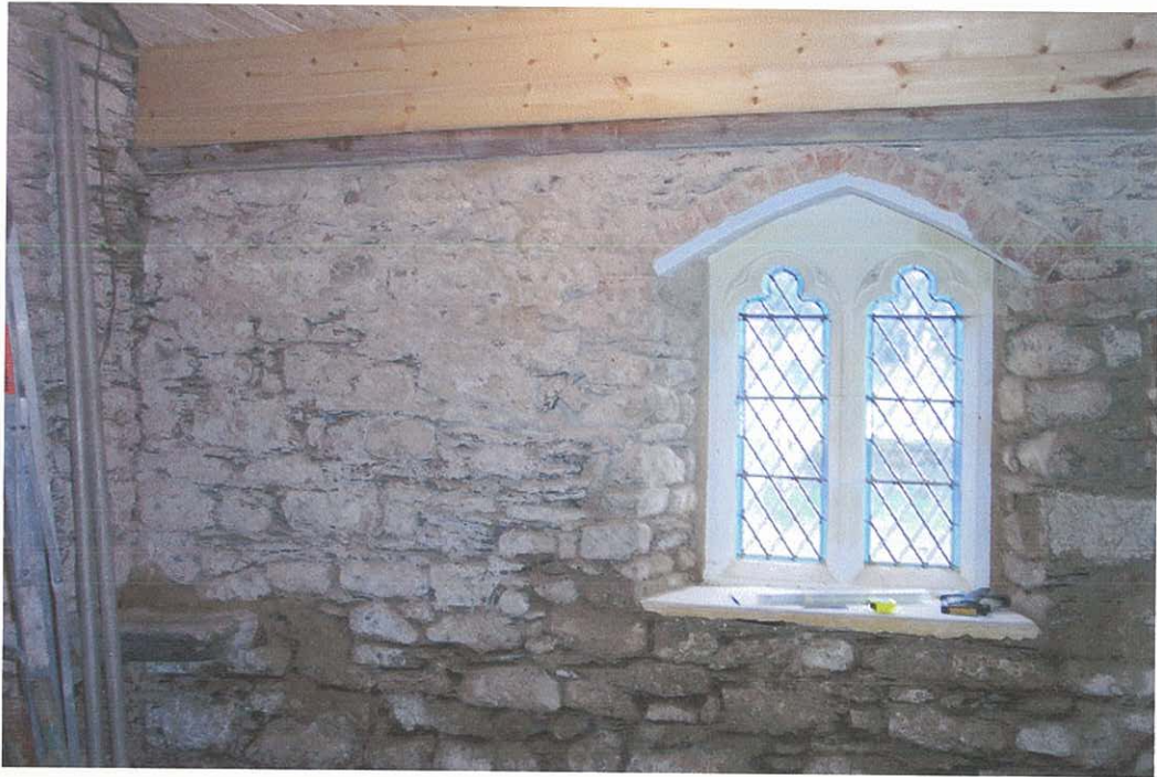
Photo 1: The east end of the south aisle wall showing the area of surviving painted plaster at the top of the wall, to the left of the window.
