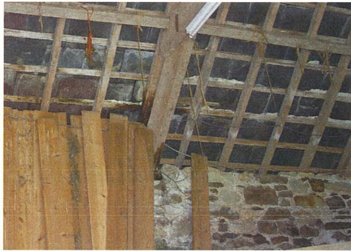
Plate 2-Rot has become established at the base of one of the roof trusses.
