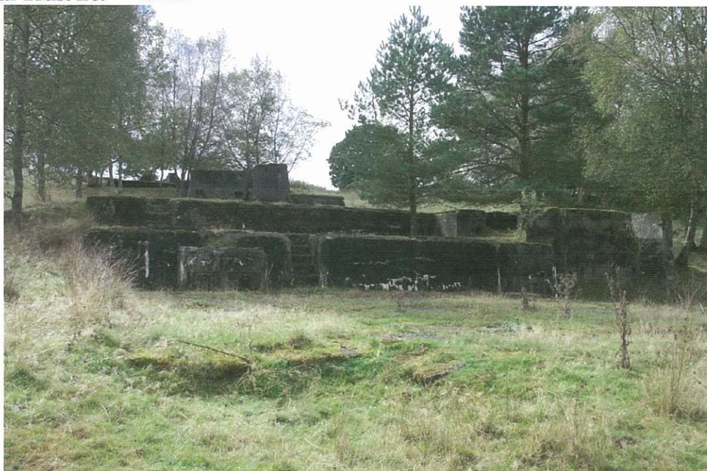
Plate 5 Concrete footings and plinths for machinery – all that remains of the final stage of ore processing at the British Goldfields processing mill (PRN 20429). These are the foundations of the ball mill (PRN 49152)
