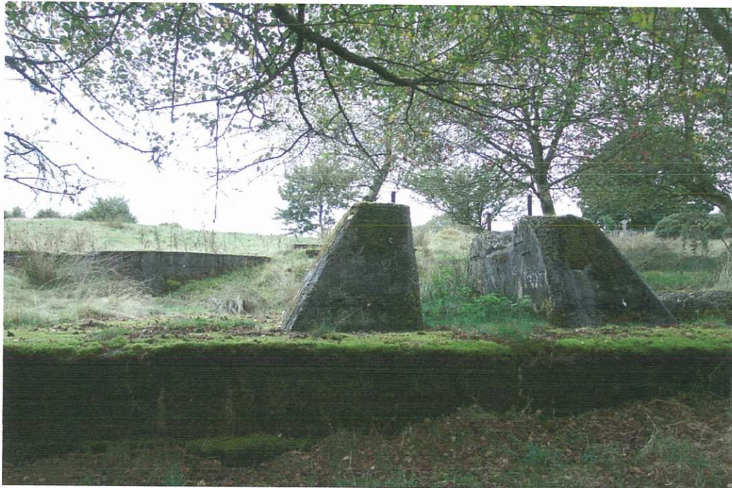
Plate 7 The concrete supports for the gyratory crusher (PRN 49154).
