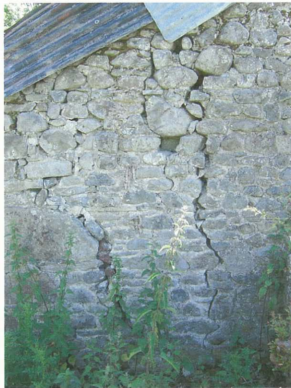
Plate 4. The north gable of the mill shows serious structural cracks which need to be monitored.
