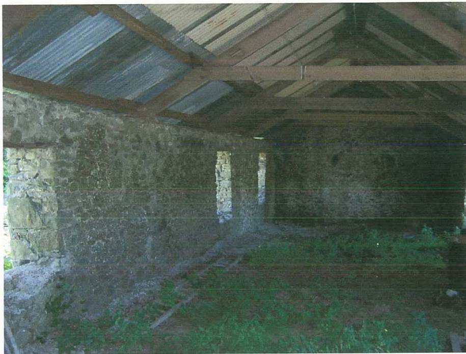
Plate 2. View of the interior of Abersannan Woollen Mill. There is a fourth window, now blocked, in this east wall. The lintels above the windows and doors have been added by the current landowner, using timbers from the collapsed roof.
