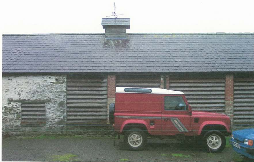
Plate 7: The east elevation of the combination farm building (PRN 48059). To the right of the picture are the wooden slat sides of the granary. To the left, the stone wall of the threshing barn. These stand above a cartshed (later used as a cowshed) which is terraced into the hillside and accessed from the west side. The small 'turret' and the weathercock are decorative finishing features, typical of this kind of well-designed estate farm.
