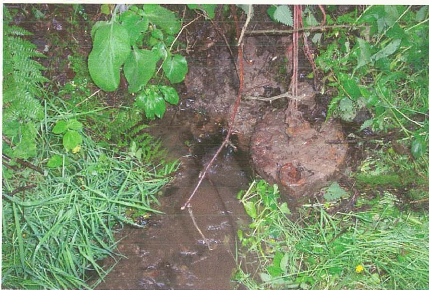
Plate 9: The iron plug which controls the flow of water from the pond (PRN 48062) into a culvert which runs under Troed y Bryn farmstead.
