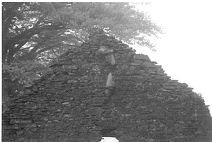
Plate 2: The west gable of Pant Gwyn cottage site (PRN 48053). The clay pipe bracketed to the wall would have acted as a flue for a grate or stove.
