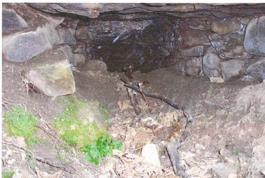
Plate 8- looking down the stone flue towards the drying chamber of corn drying kiln (PRN 48295).
