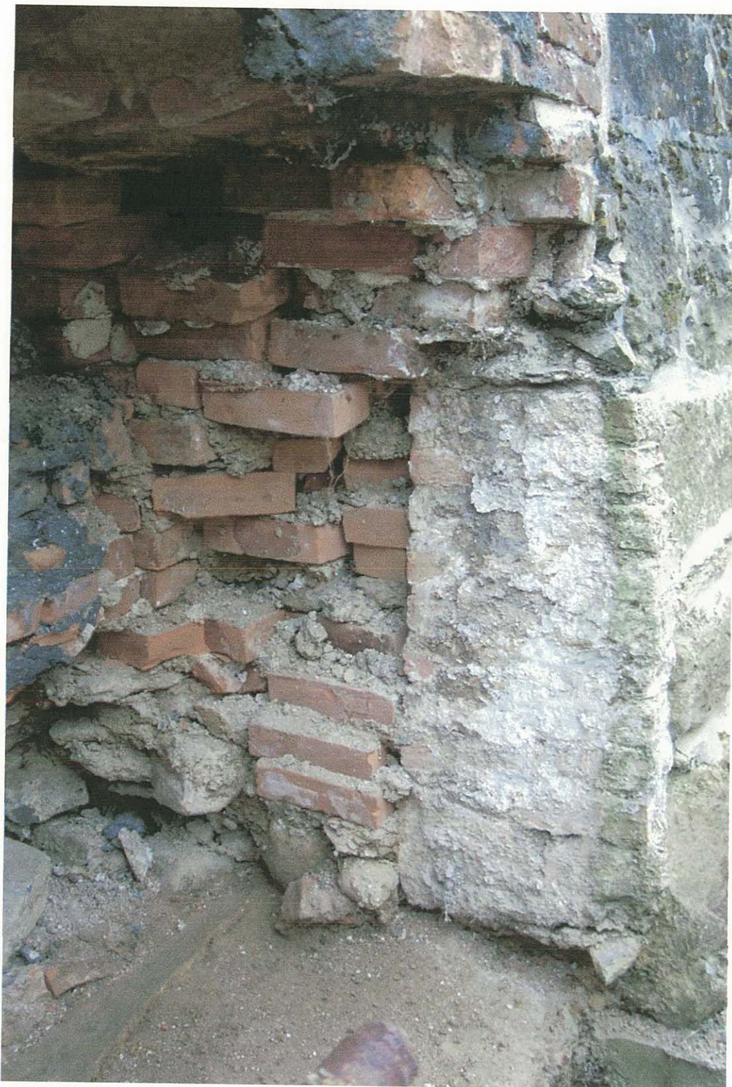
Plate 6: West side of the crypt entrance (right) with brick blocking (left)
