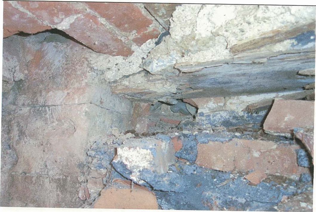
Plate 2: Dressed limestone medieval door Jamb (left), brick vault (above) and brickwork blocking the entrance to the crypt
