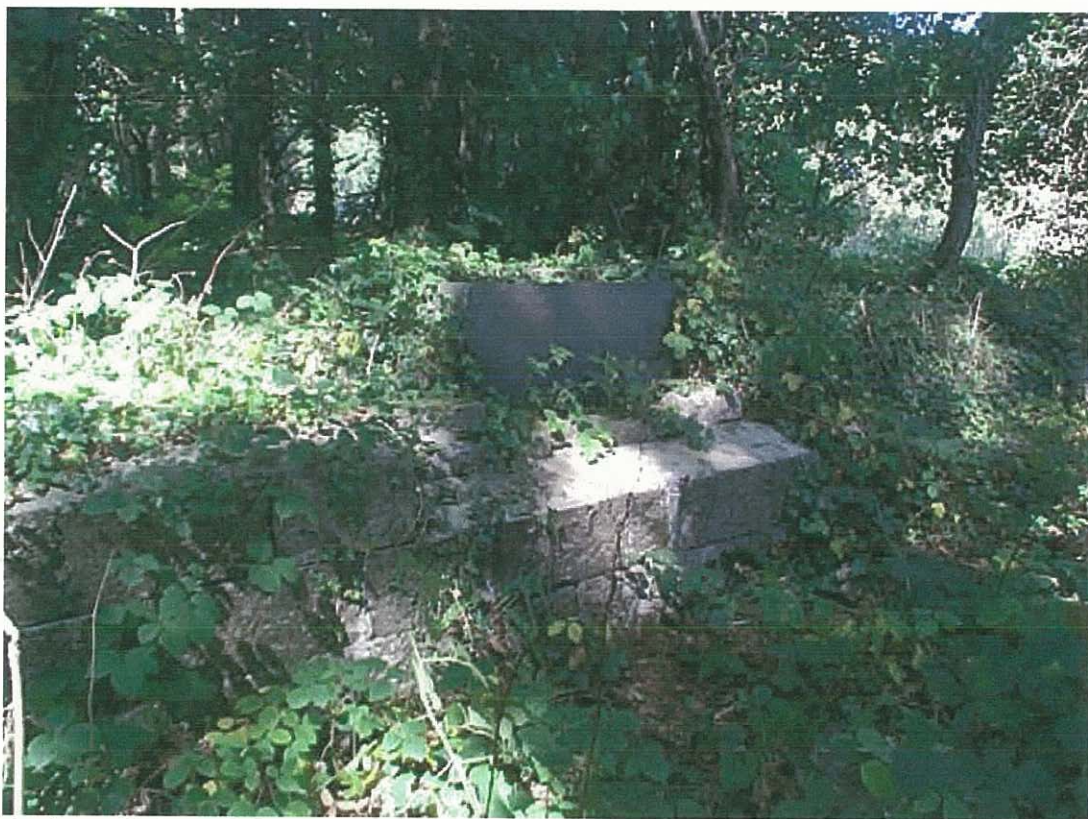
Plate 9. A small slate-slab water cistern set into the walls of the sunken garden (PRN 48637). The water ran through a system of pipes to feed a central pond.
