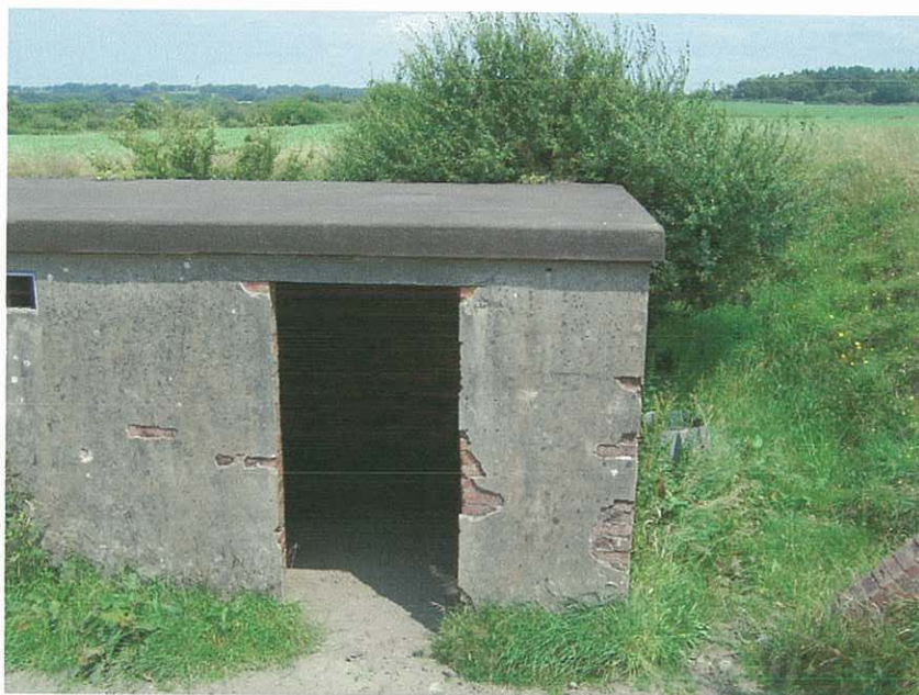
Plate 5. Incendiary store (PRN 48632). Although some vegetation is beginning to colonise the building, the earthwork enclosure around it is well preserved and the building itself is stable.
