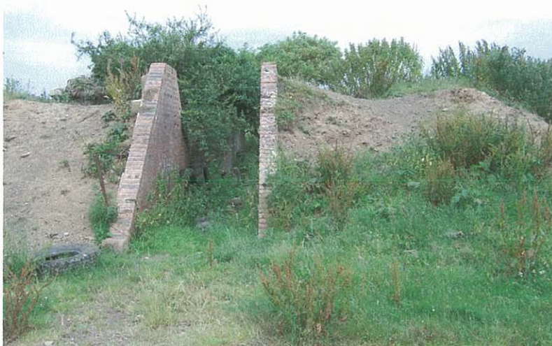
Plate 3. A brick supported entrance through the blast wall which surrounds a bomb store (PRN 48628). The building itself is behind the vegetation, just to the left of the entrance.
