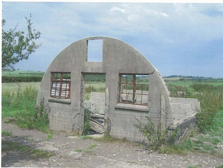
Plate 4. The remains of a military building (PRN 48629). This building would have had an arched corrugated metal roof – the walls and gable stand to their full height.
