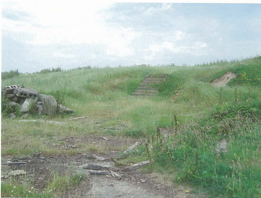
Plate 2. The remains of a bomb or incendiary store (PRN 48627). The embankment around the site is clearly seen, with the flight of steps surviving on its north side. The building foundations are in the foreground and to the right of the picture.
