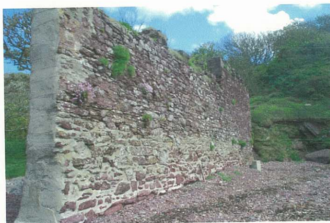
Plate 6: The west section of the sea wall (PRN 34759). The cement render on the surface at the forefront of the picture was applied by a Manpower Services team, when they repaired the central gap in the wall.
