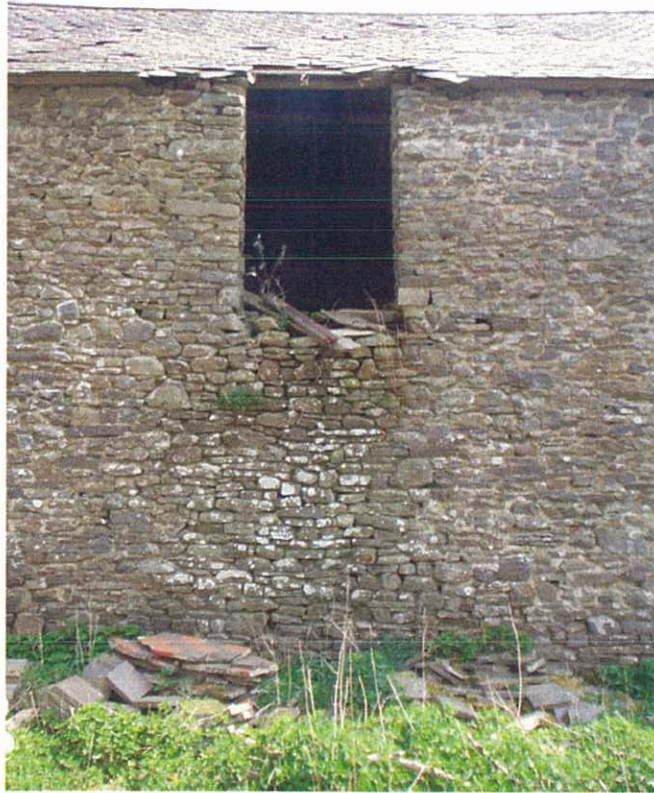
Plate 6- water damage to masonry bonds in the building range at Tir Bach (PRN 47902)
