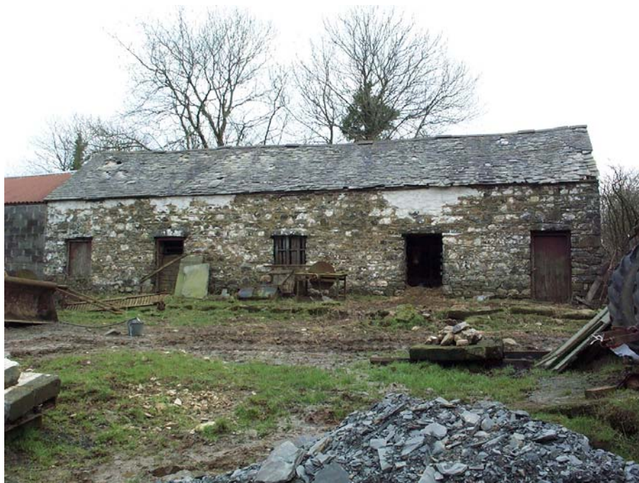
This cow shed is a fine example of its type with an original slate roof, pegged with wooden dowels
