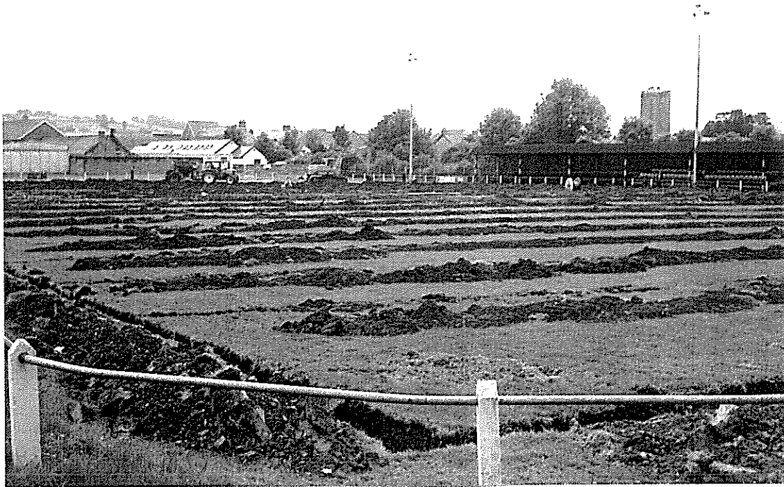
Fig. 5 Carmarthen Richmond Park: Two views of the 1998 drainage trenches showing their extent and method of mechanical excavation.
