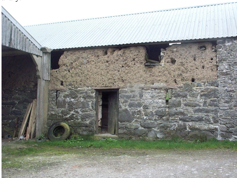
PRN 44871 the central section of the building showing the clom wall to the loft. The vent loops on the ground floor have been adapted from larger openings. The break between the central section and northwest section of the building (to the right) is clearly visible.
