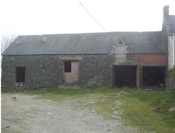
PRN 44865 18 th century threshing barn showing cart openings and central winnowing door
