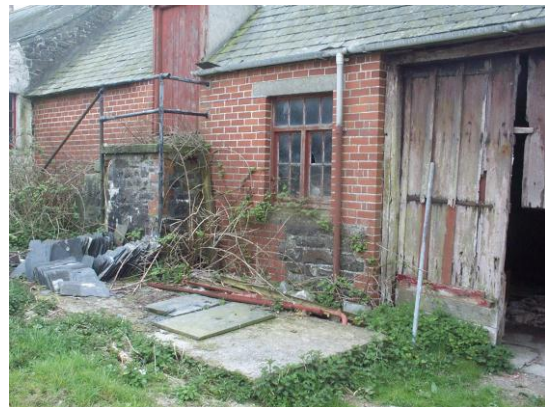
PRN 44865 wheel pit capped with concrete in 1961. Note the extensive rebuilding.
