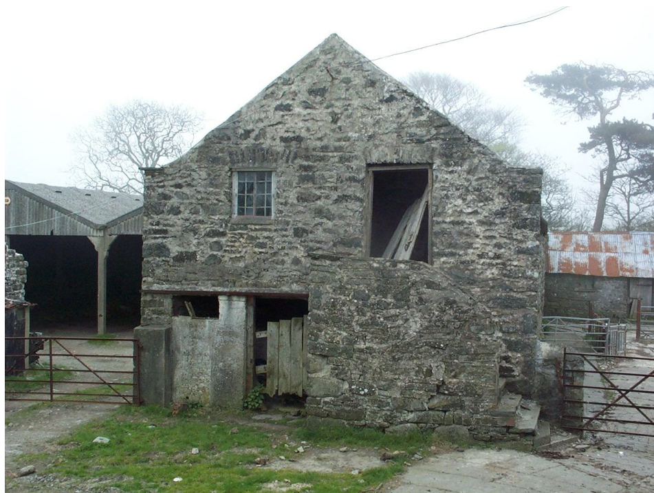
PRN 44871 the northwest gable wall of building showing blocked cart opening and stone steps to first floor granary.
