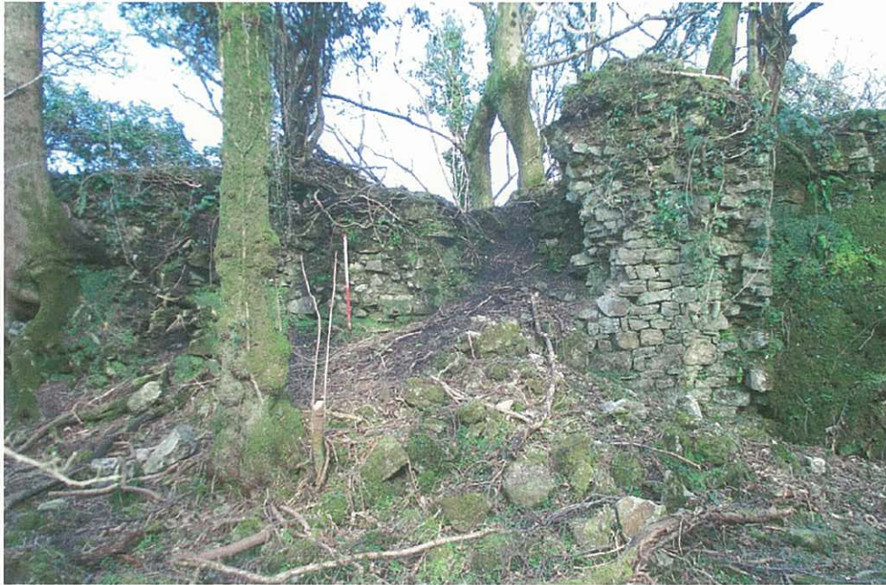
Plate 9: Llandyfan Old Forge (PRN 44441). The blocked opening in the dam. The function of this feature remains unclear. It may be a blocked sluice, but only excavation could elucidate this further.
