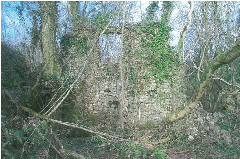
Plate 14: Llandyfan New Forge (PRN 44446). View across the wheelpit area towards the southwest gable wall. The water fed an overshot wheel from a launder that was originally in the area now occupied by the large tree to the left of the wall.
