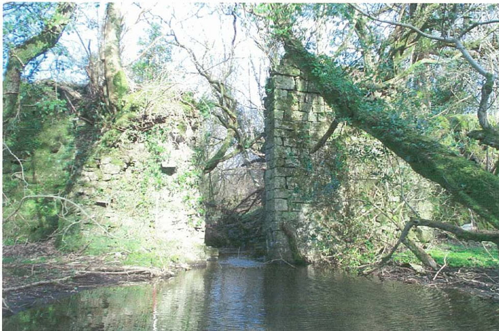
Plate 2: Llandyfan Old Forge (PRN 44441). The sluice exit in the dam. Note the ponding in front of the dam, which is leading to increased waterlogging of the central section of the site.
