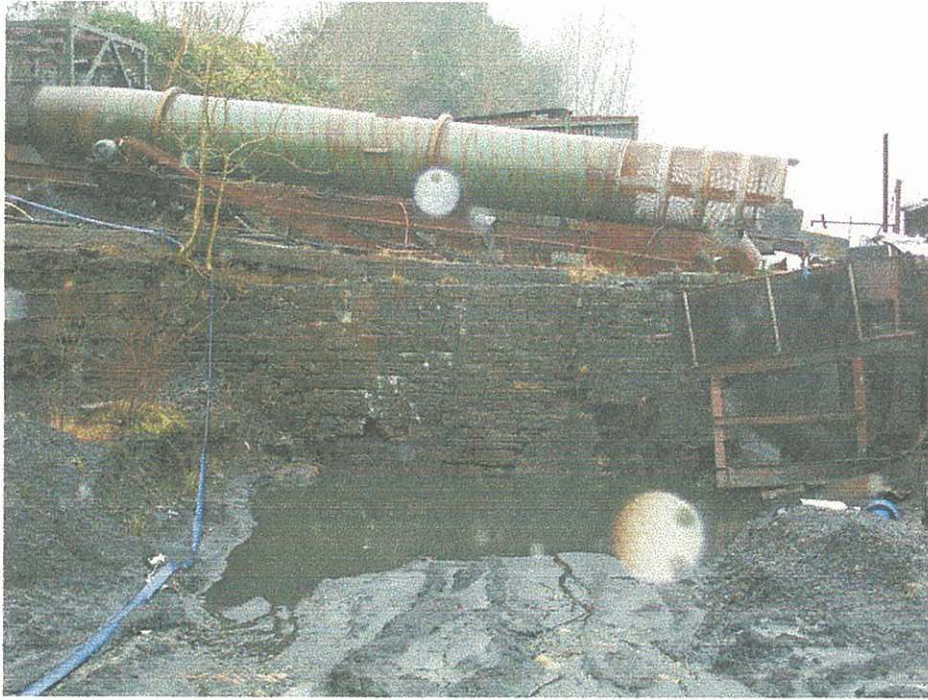
Plate 1: Remains of the brickworks building constructed on the site of the old furnaces and now incorporated into the base for the washery conveyor.
