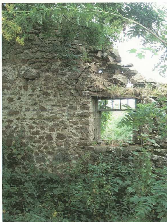
Plate 2 – decayed lintel and stonework above
