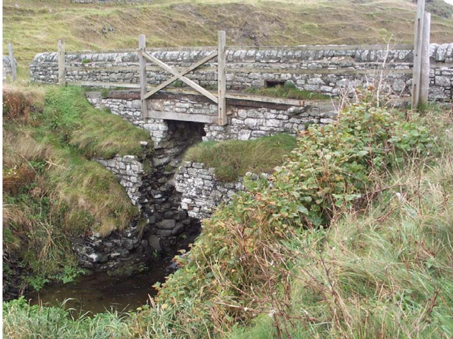
Prn 48732 – the upper level of this dam supports the public footpath, below the stone revetment has been breached in the centre.
