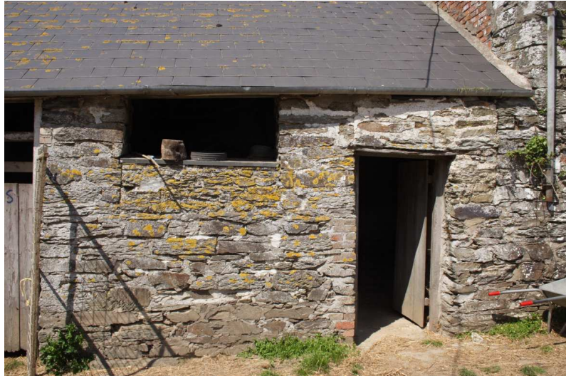
The lower part of the range. The filled in remains of former openings are visible in the walls.
